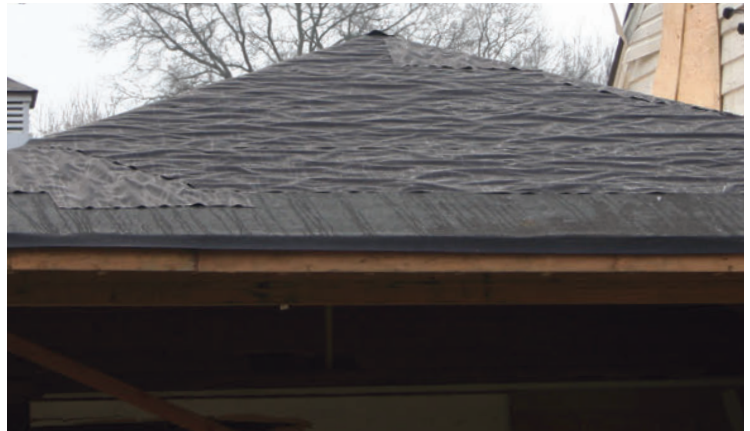
Conventional organic felts can absorb moisture, causing severe buckling and wrinkling—and a terrible-looking roof
